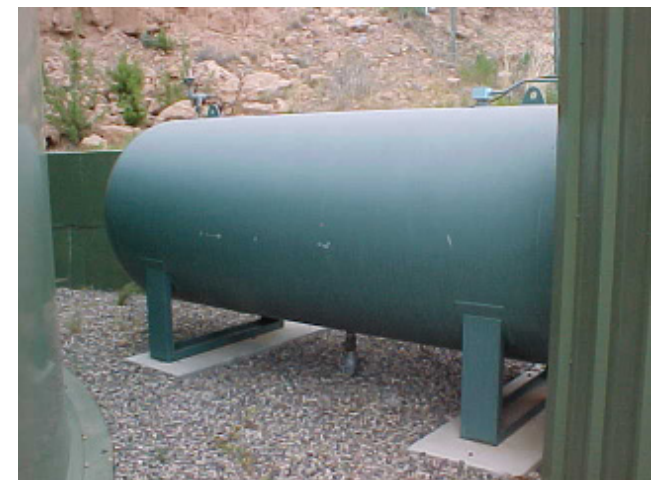
A Metal Storage Tank
