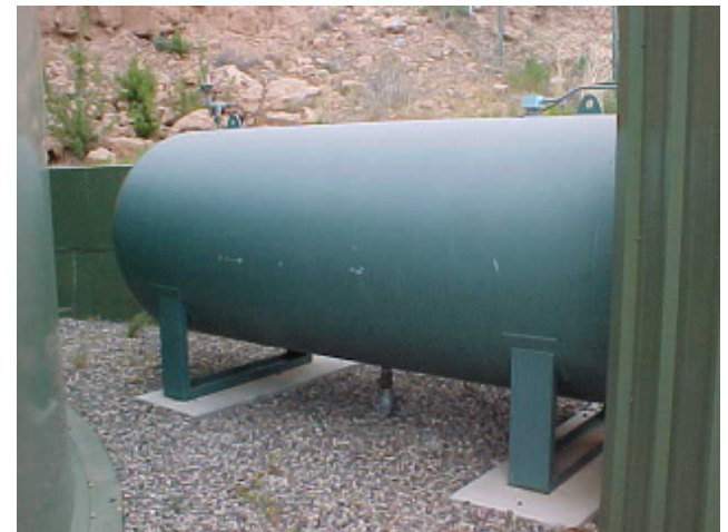
A Metal Storage Tank
